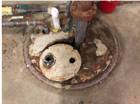
5. Sump pit in mechanical room by men's locker room (Permit Required)
