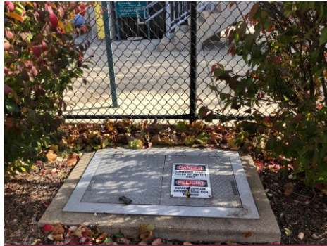
4. Collector tank for spray ground (Permit Required)
