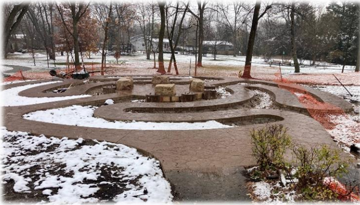
Newly poured stamped concrete
