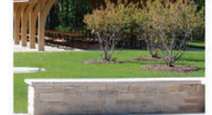
Existing Factory Wall with New Limestone Facade and Cap
