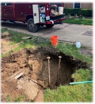
The water supply line to the greenhouse has been replaced. About 200' of polyethylene line was directionally bored from the city main located near the tennis courts. The old line was in excess of fifty years old in some areas.
