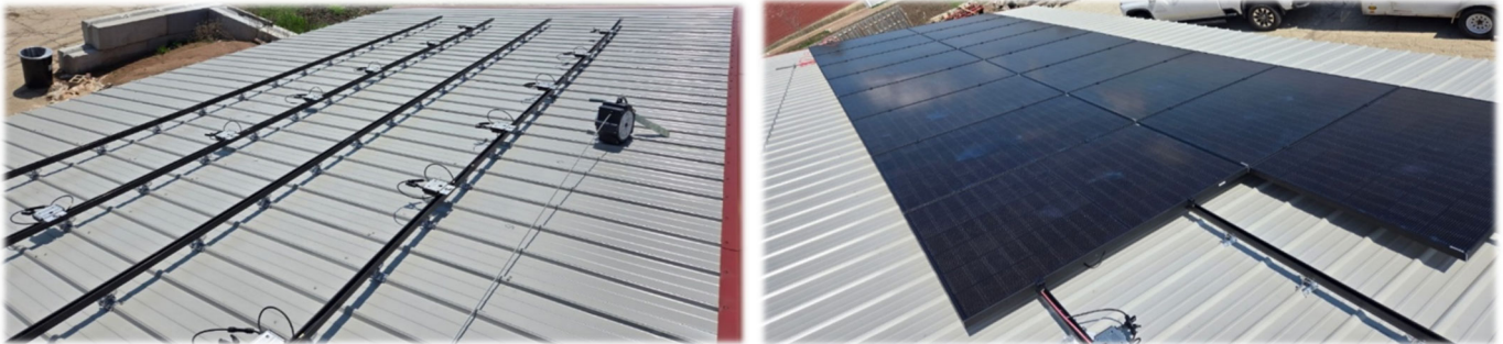
Mounting brackets were installed on the roof of the barn, soon to be followed by the solar panels themselves.
