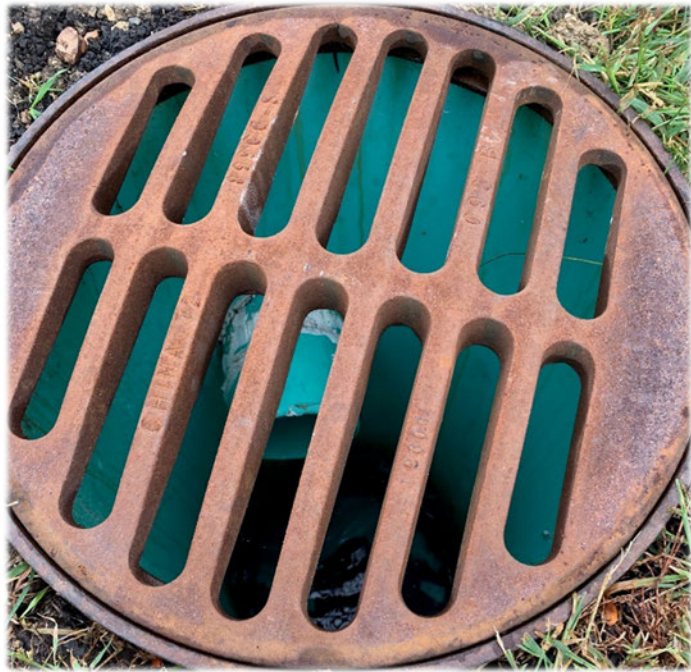
Water moves by pipe to a nearby catch basin
