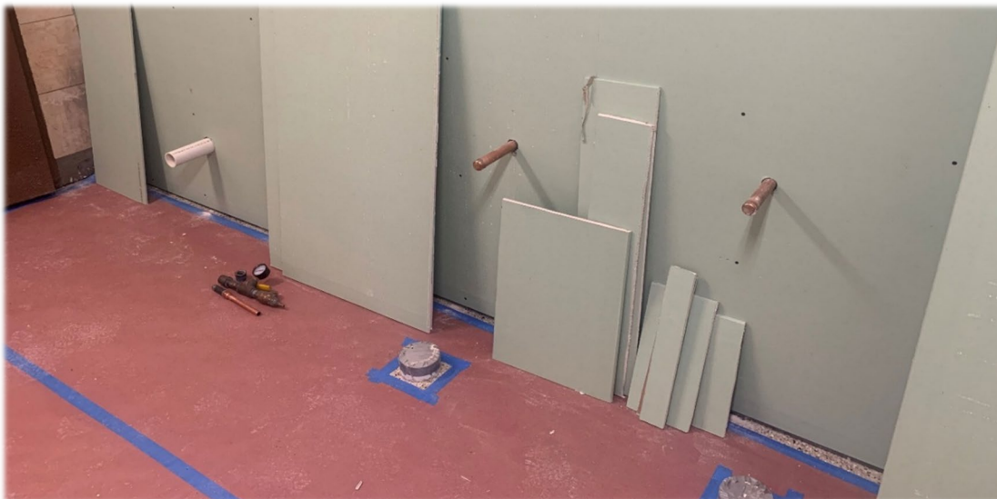
Newly installed moisture resistant drywall and epoxy coated floors (covered by paper during construction)
