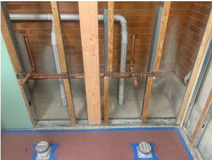
Reconstructed walls will hide a new plumbing chase
