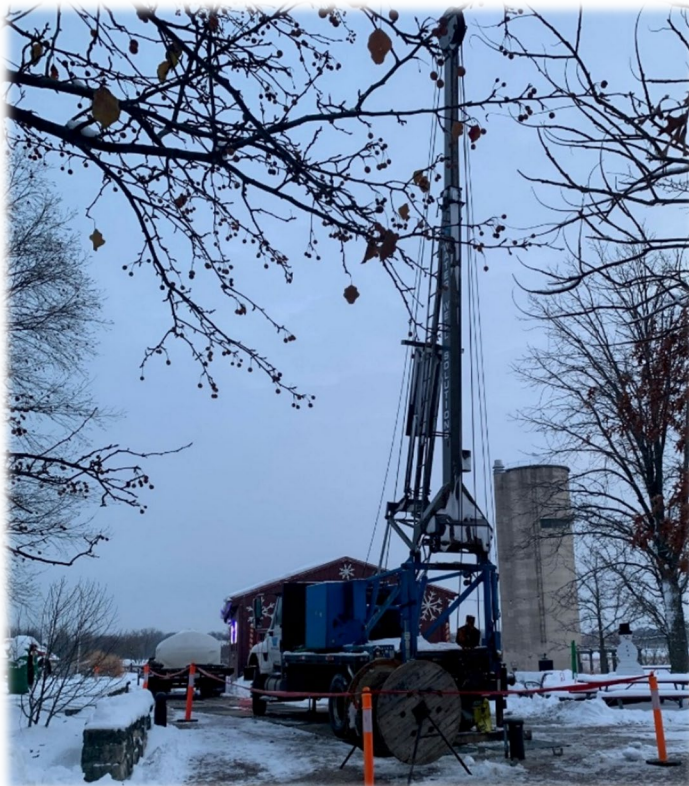
A well drilling rig is used to pull out the old pipe and pump
